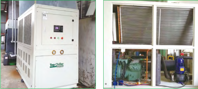
30HP 菲律宾风冷低温机 AIR COOLED GLYCOL CHILLER IN PHILIPPINES
