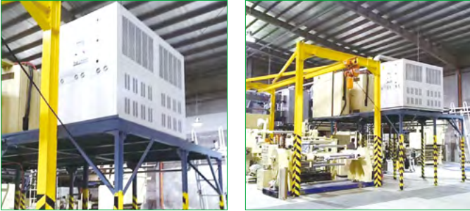
30TON 菲律宾风冷机组 AIR COOLED CHILLER IN PHILIPPINES
